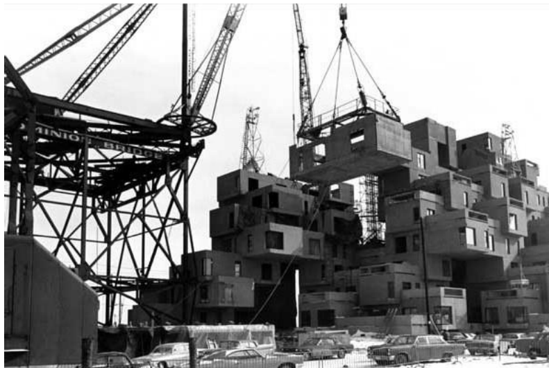
Figure 40: Site Construction. Source: Google
